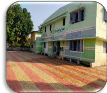
Paver block installation carried out at Shantiniketan Vidhyalay near Sayakha Plant.
