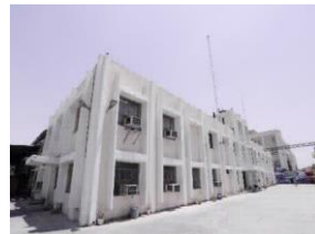
RFL I & II - Bahadurgarh
