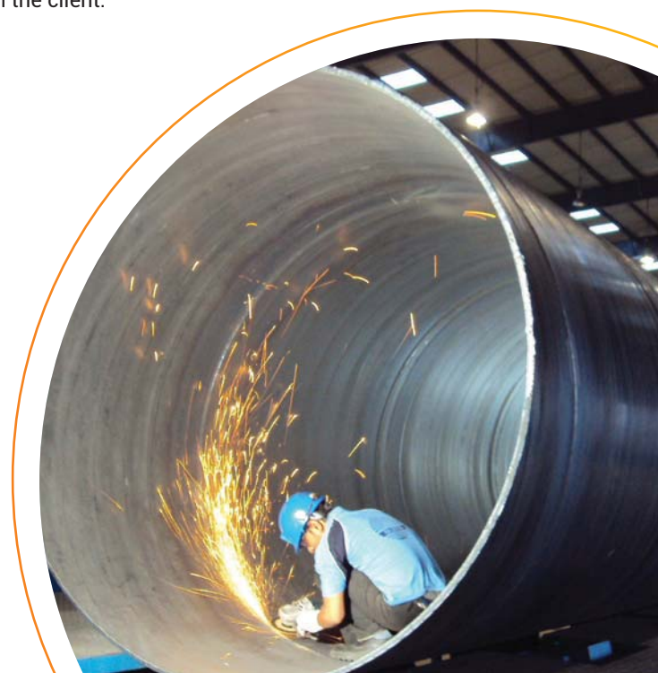
Spiral Pipes at Anjar Plant, Gujarat
