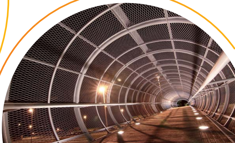
Tube railway infrastructure
