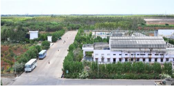
Greenery around plant
