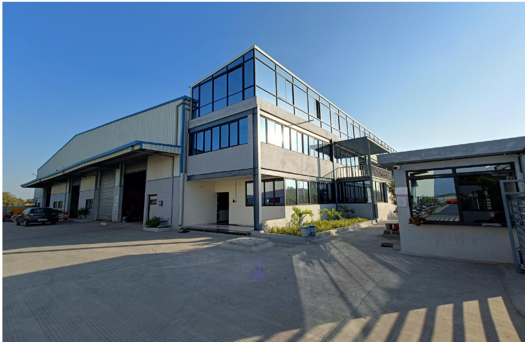
Advait Infratech – ACS Plant at Kadi, Mehsana, Gujarat
