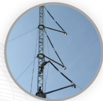
Emergency Restoration Systems (ERS) Supply and Installation
