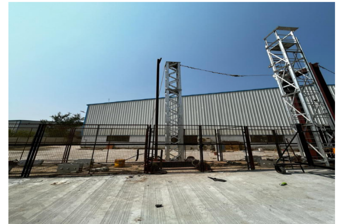
Advait Infratech ERS Testing Station – Ahmedabad, Gujarat
