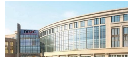
NMC Speciality hospital, Abu Dhabi
