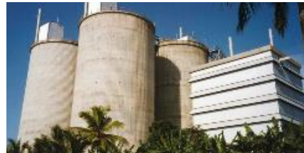
Bulk Cement Terminal, Colombo
