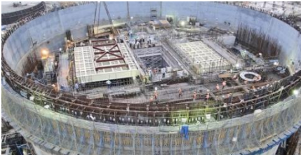
Kakrapar Nuclear Power Plant, Guj
