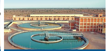
Water Treatment Plant, Barmer
