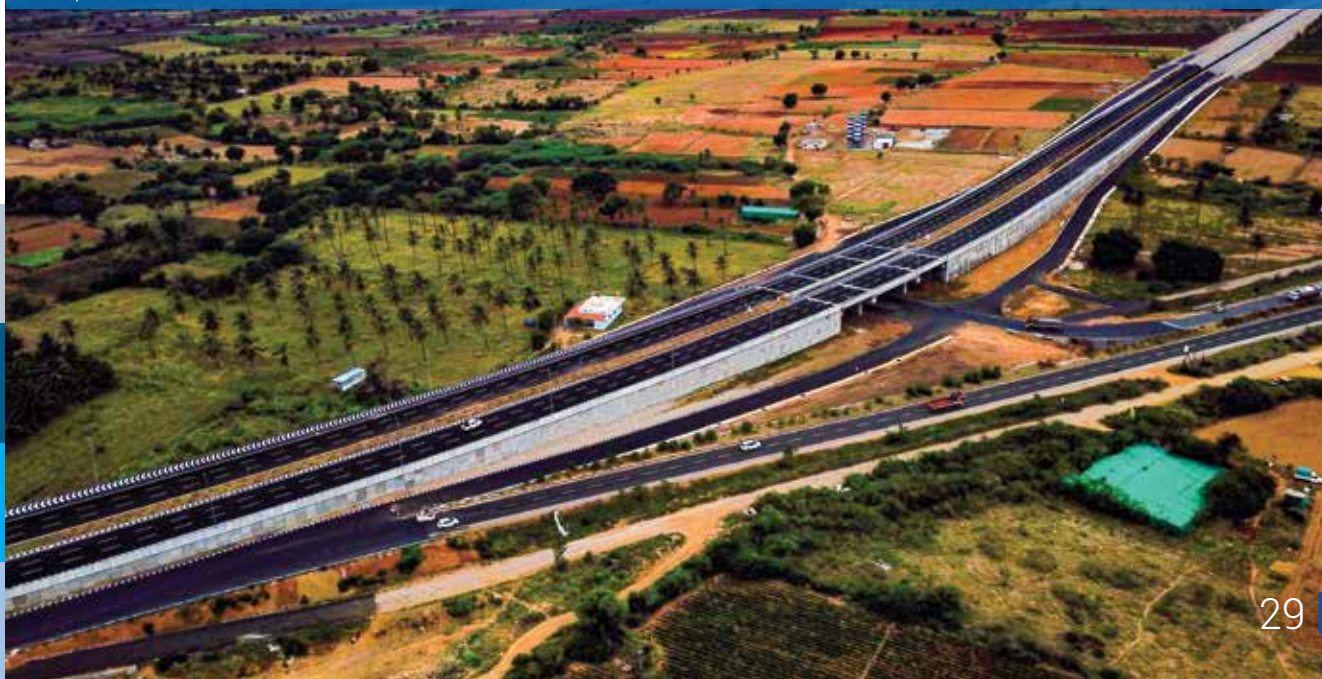
Flyover at 0+550 under 6-Laning of Chitradurga – Davanagere including Chitradurga bypass from Km 0+0 to Km 20.7 & Km 208 to Km 260 of NH-44 (Old NH-4) in the state of Karnataka
