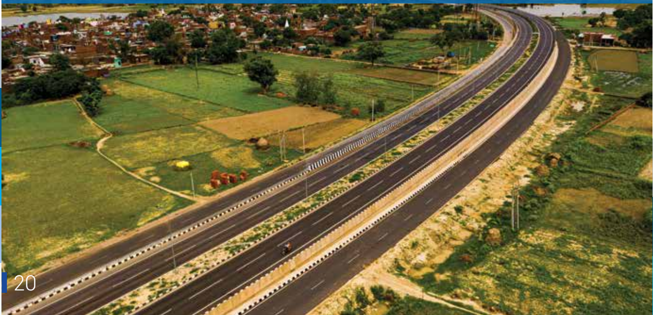
Pilua Bypass at Km 202+465 under Four Laning of Aligarh – Kanpur section package-II from Bhadwas to Kalyanpur of NH-91 in the State of Uttar Pradesh under Bharatmala Pariyojana
