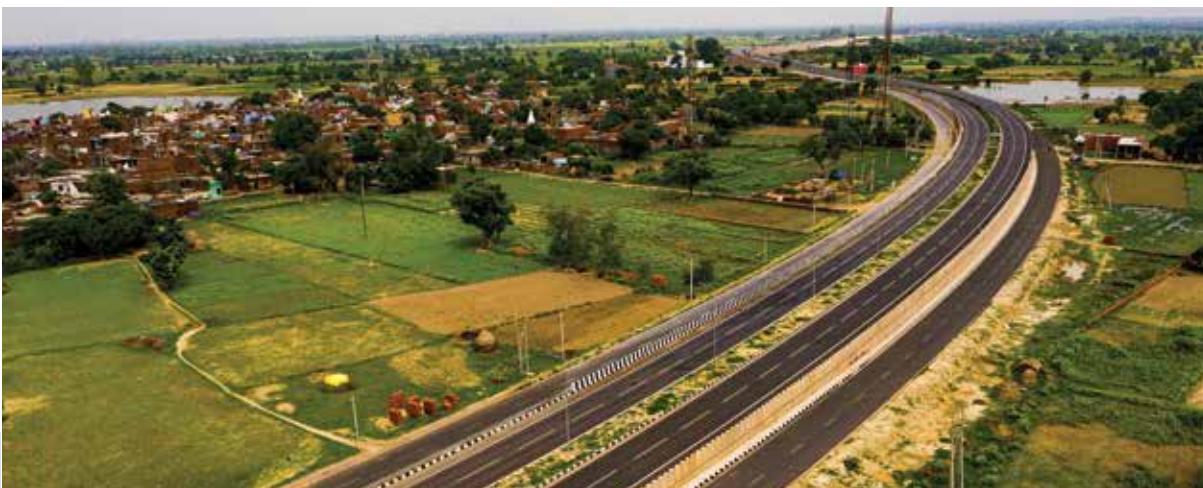
Pilua Bypass at Km 202+465 under Four Laning of Allgarh – Kanpur section package-II from Bhadwas to Kalyanpur of NH-91 in the State of Uttar Pradesh under Bharatmala pariyojana
