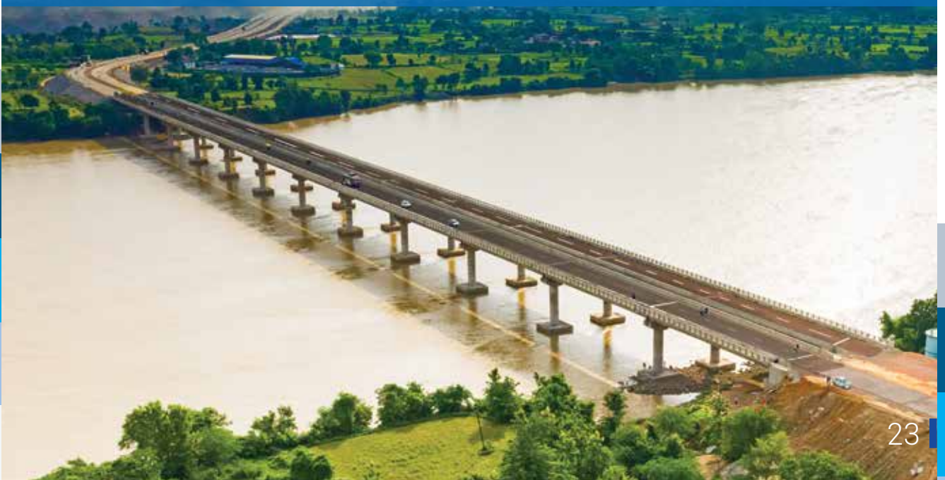
Four lane Major Bridge on Betwa River under Four laning of Jhansi-Khajuraho section (Pkg –I) from km 0.0 to km 76.3 of NH-75/76 in the state of UP & MP under NHDP Phase-III
