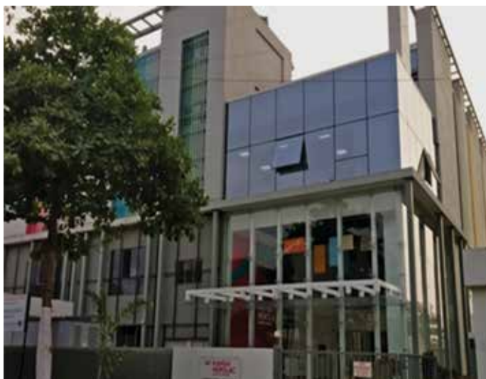
New R&D Facility
