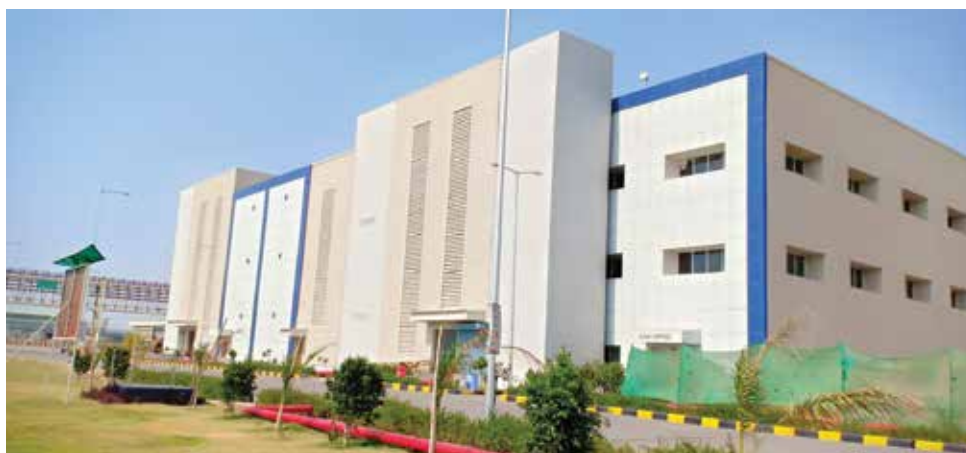
State-of-the-art plant at Sayakha, Gujarat
