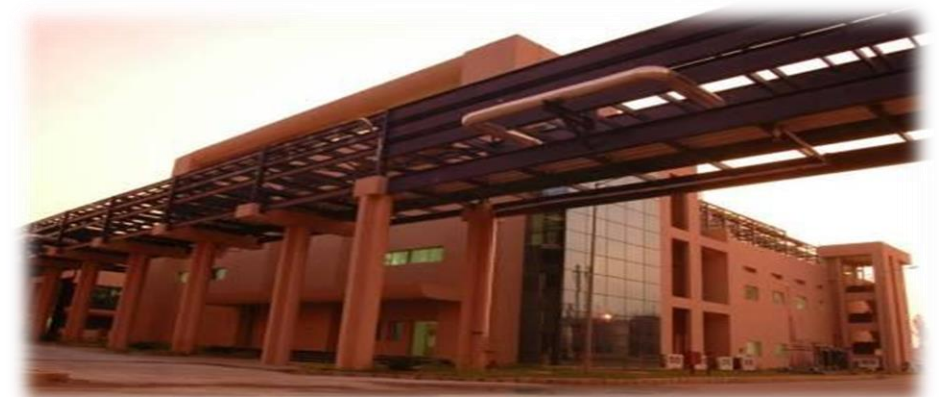
Syngene's USFDA approved manufacturing facility at Bangalore
