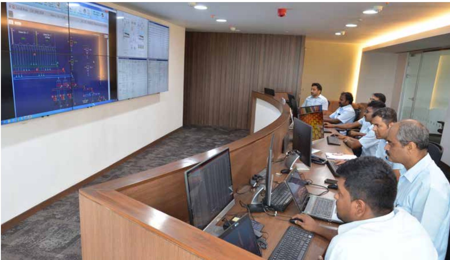
Tracking of operations of the Units from the Corporate Office
