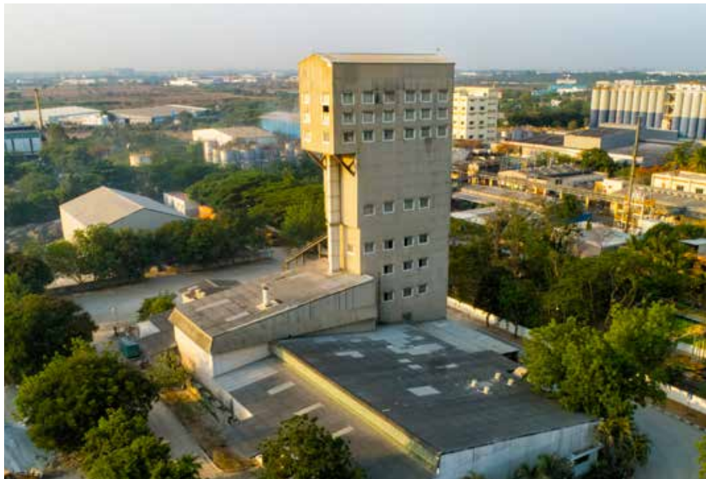
Dry-mix Unit, Sriperumbudur, Chennai
