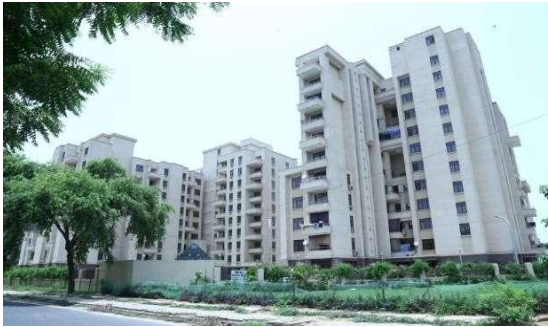
Residential accommodation for NHA staff at Sector 17, Dwarka, New Delhi
