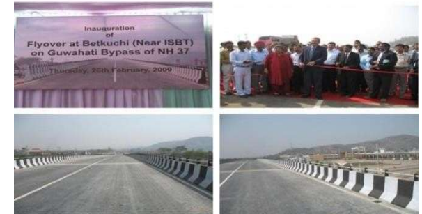
Construction of 2 lane flyover on Guwahati Bypass of NH-115 (earlier NH-37) in the state of Assam
