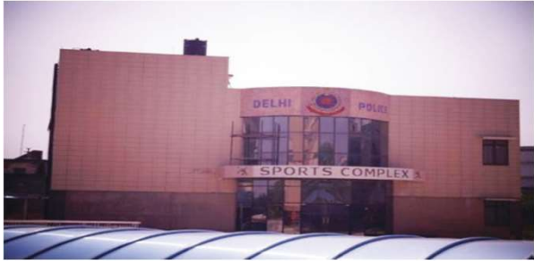
Police Station & Residential Quarters at Kondli, New Delhi for MHA, Delhi Police through RITES Ltd.
