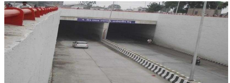
Construction of RUB at Badli, New Delhi
