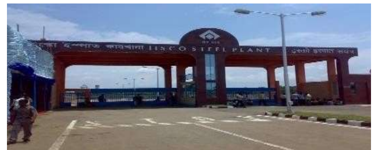
Approach road 2 lane from GT road at Neamatpur to Bumpur, West Bengal
