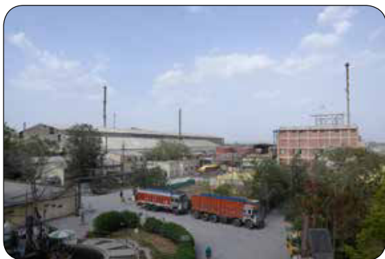
Indore Plant View
