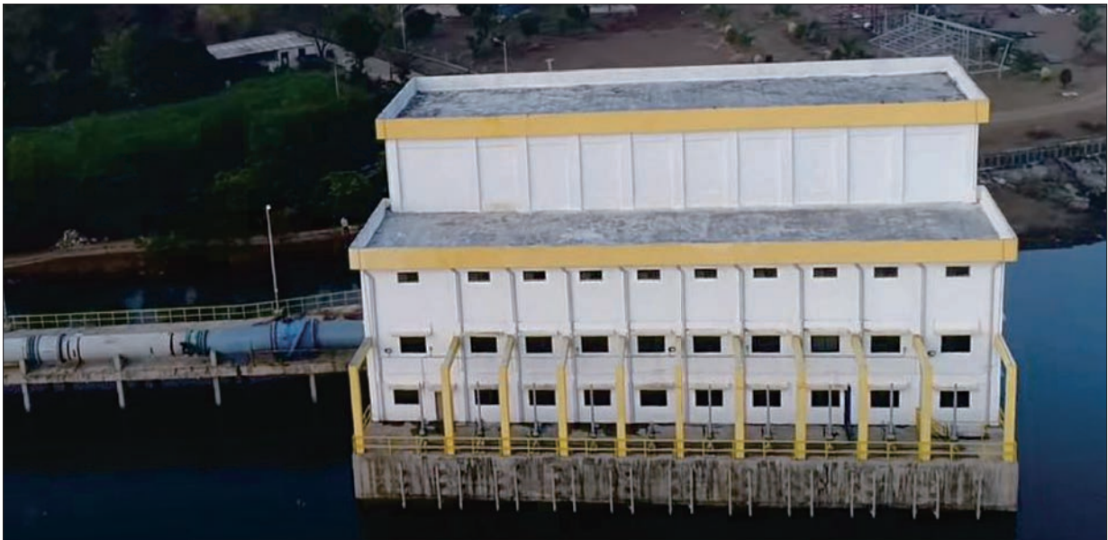
Pump House - Bhama Askhed Project, Pune
