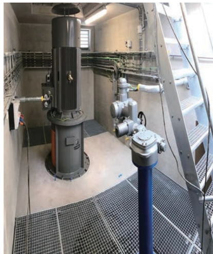
Supply of first fish-friendly Concrete Volute pump in Europe, wherein the prefabricated design was conceptualised & manufactured by Rodelta Pumps International BV
