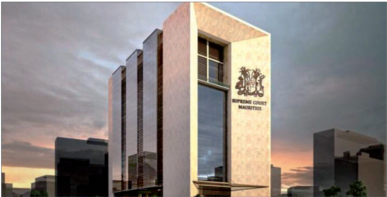
Firefighting Pumps for New Supreme Court Building, Mauritius
