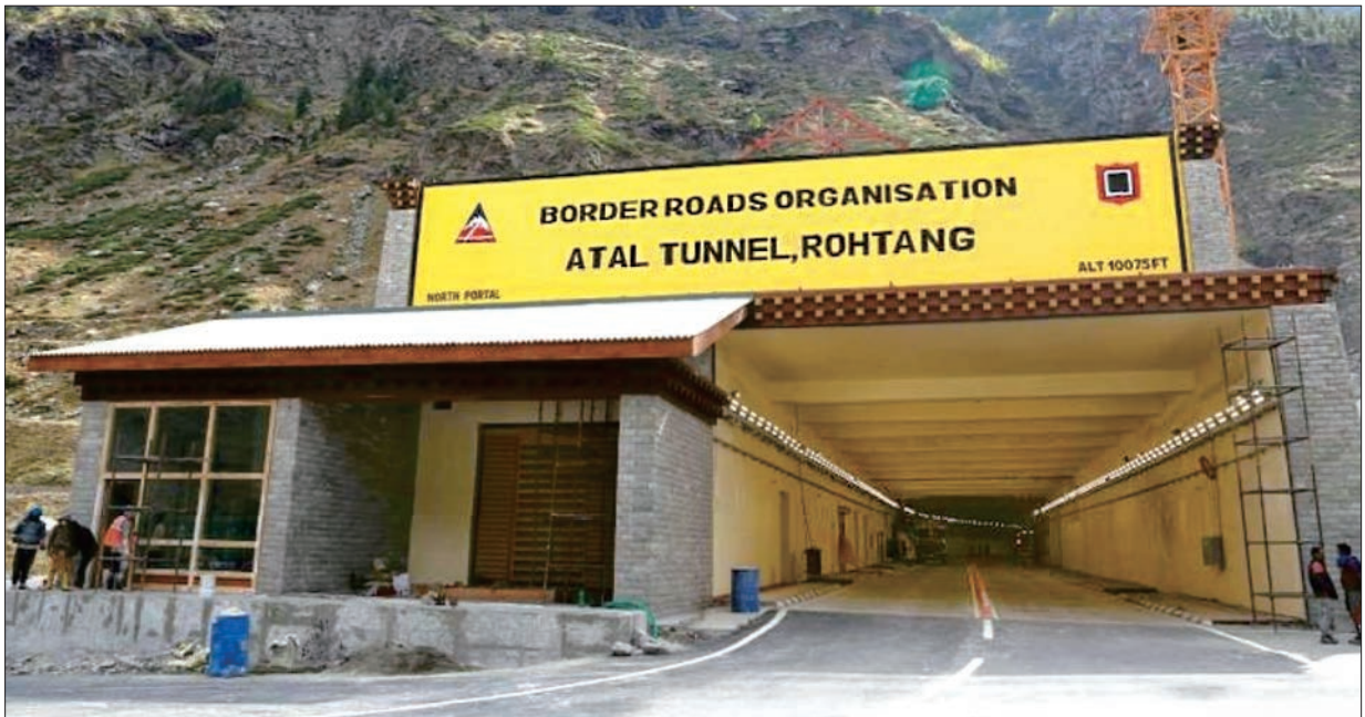
Firefighting Pumps for Atal Tunnel, Rohtang
