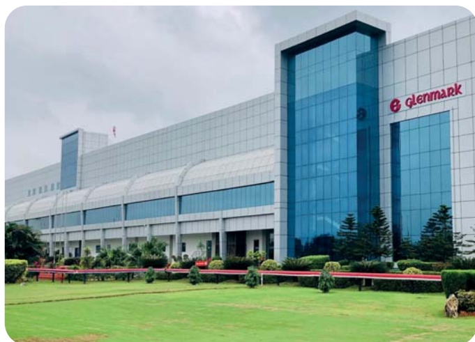
Glenmark's Indore facility in India
