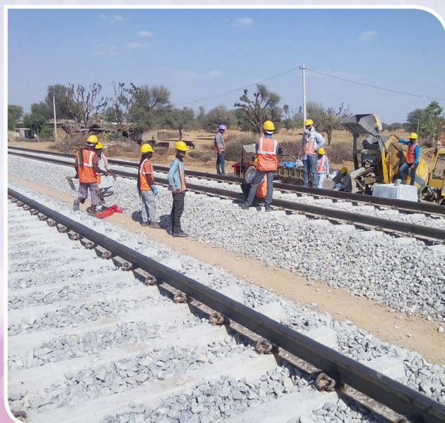
Semi-mechanised track installation
