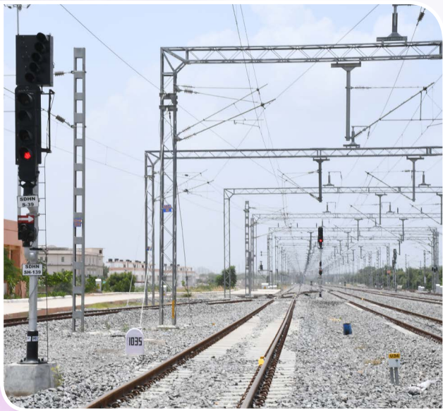
Working Signalling Gears in WDFC
