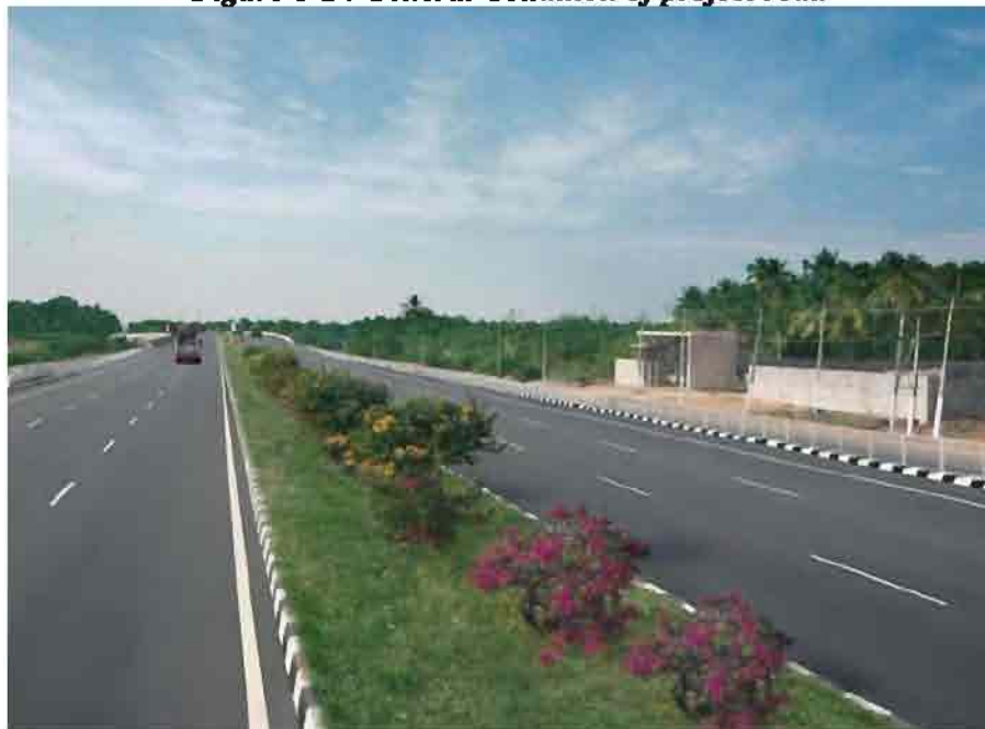
Figure 8-2 : General Condition of project road
