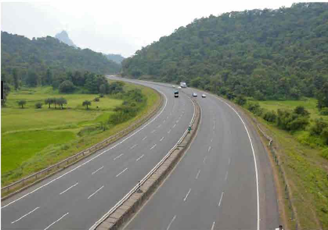
Figure 8-3 : General Condition of Project Road
