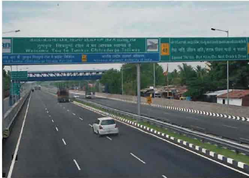
Figure 8-1 : General Condition of project road
