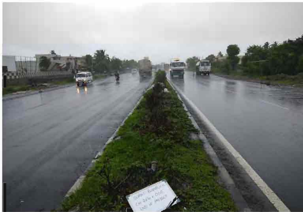
Figure 8-4 : View of Project Road
