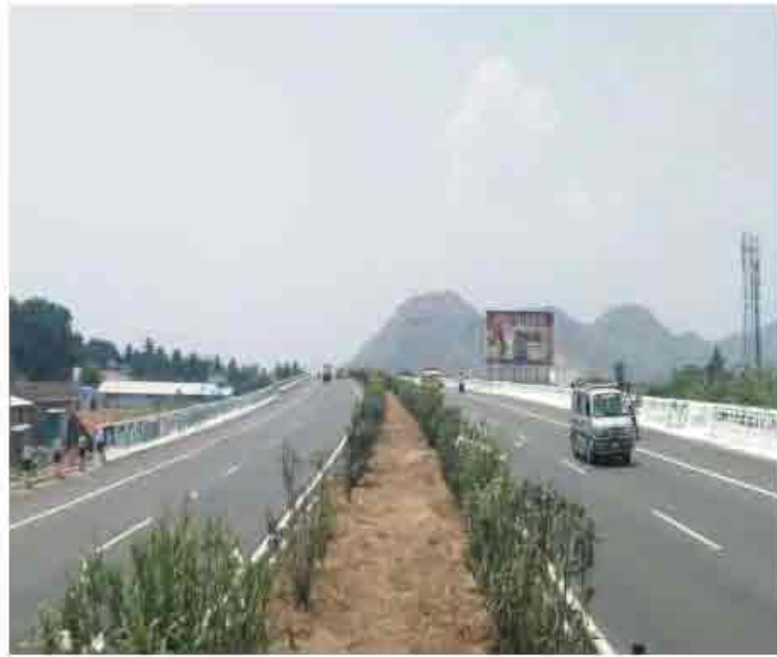
Figure 8-3 General Project Condition
