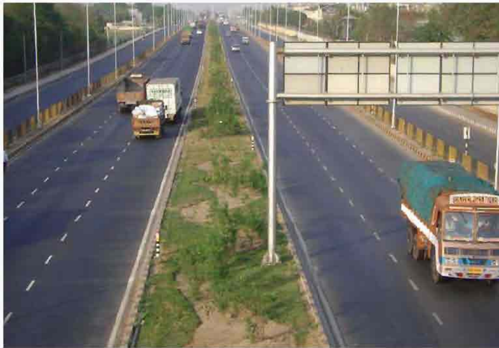
Figure 8-3 : General Condition of Project Road
