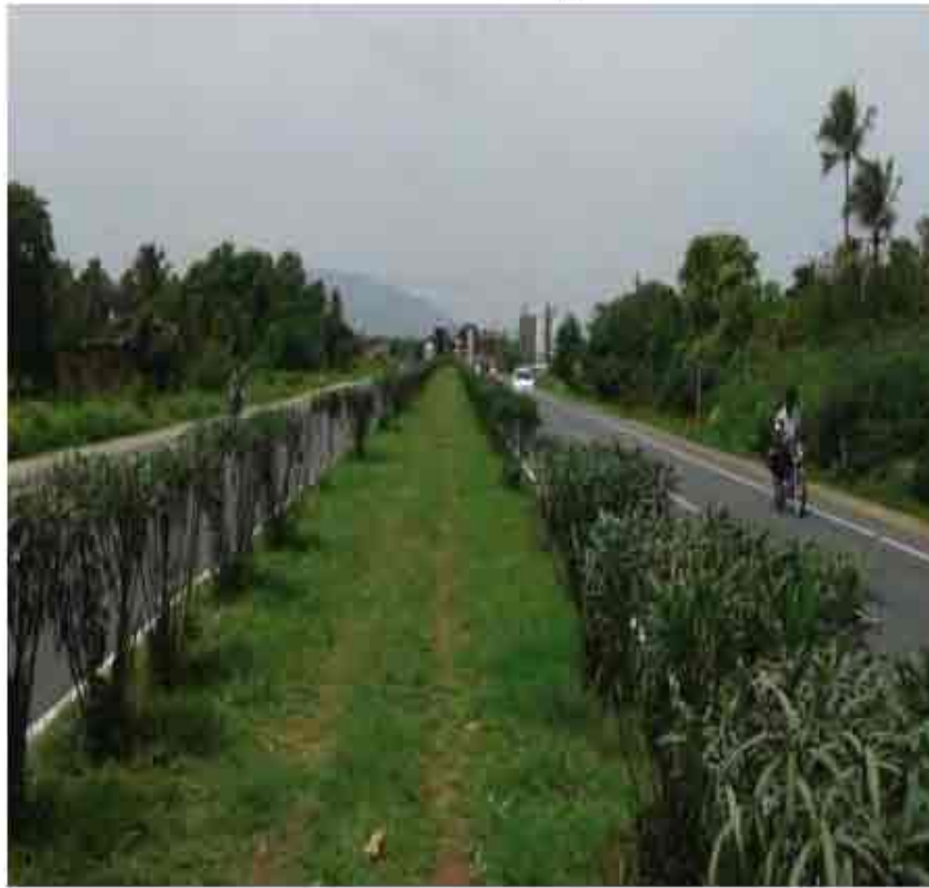
Figure 8-4 General Project Condition
