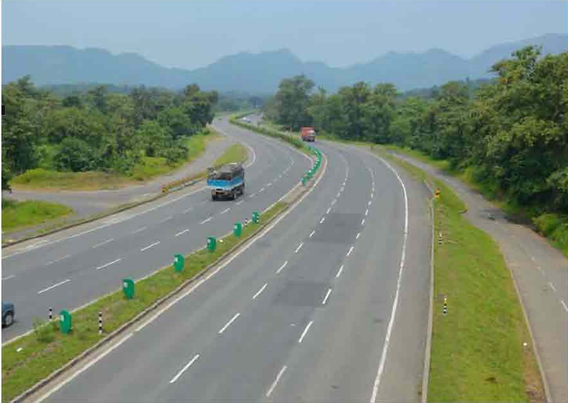
Figure 8-1 : General Condition of Project Road
