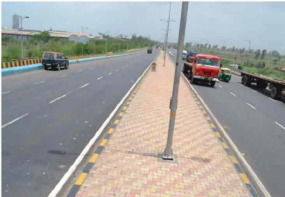
Figure 8-2 : General Condition of project road
