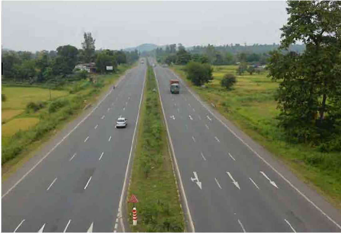
Figure 8-2 : General Condition of Project Road
