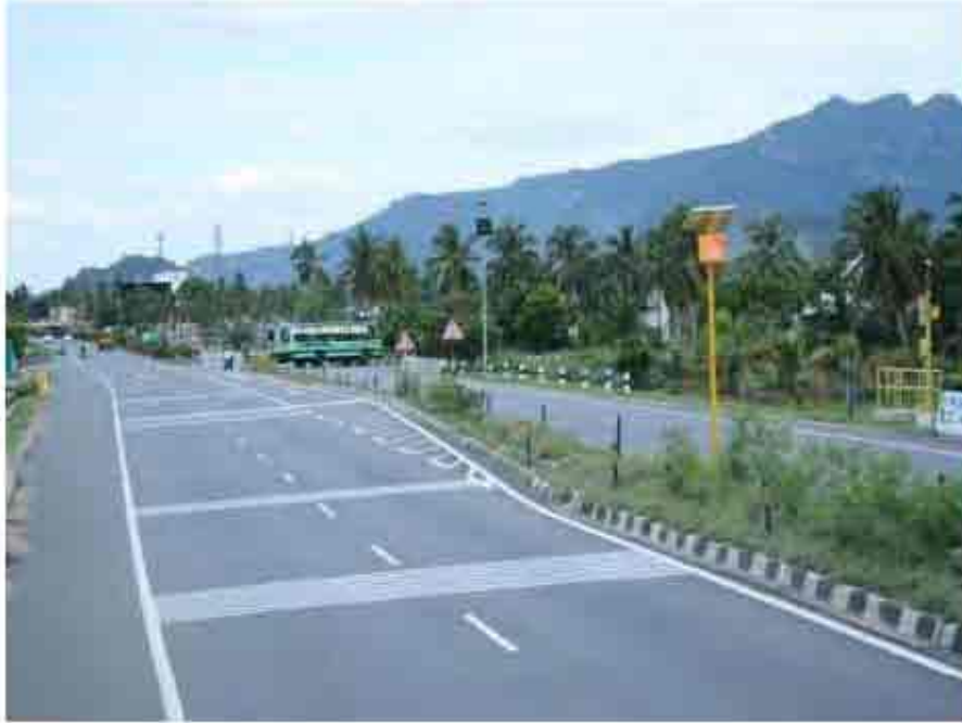
Figure 8-1 : General Project Condition
