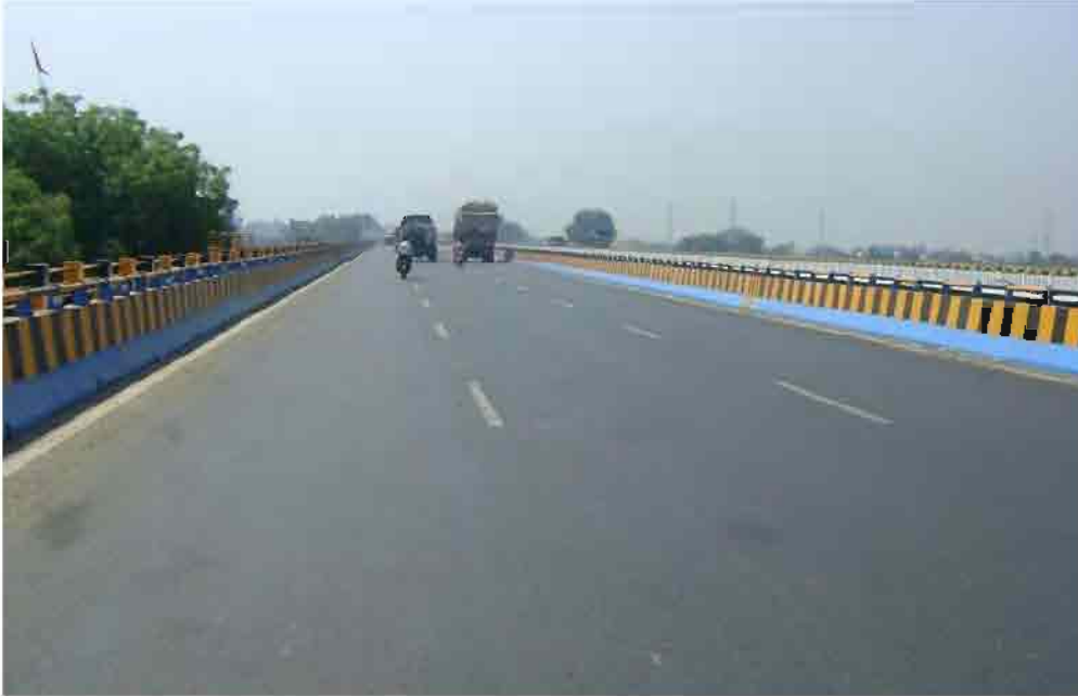
Figure 8-1 : Tapi Bridge Condition
