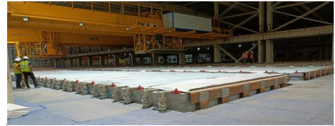
Refinery Cells commissioned
