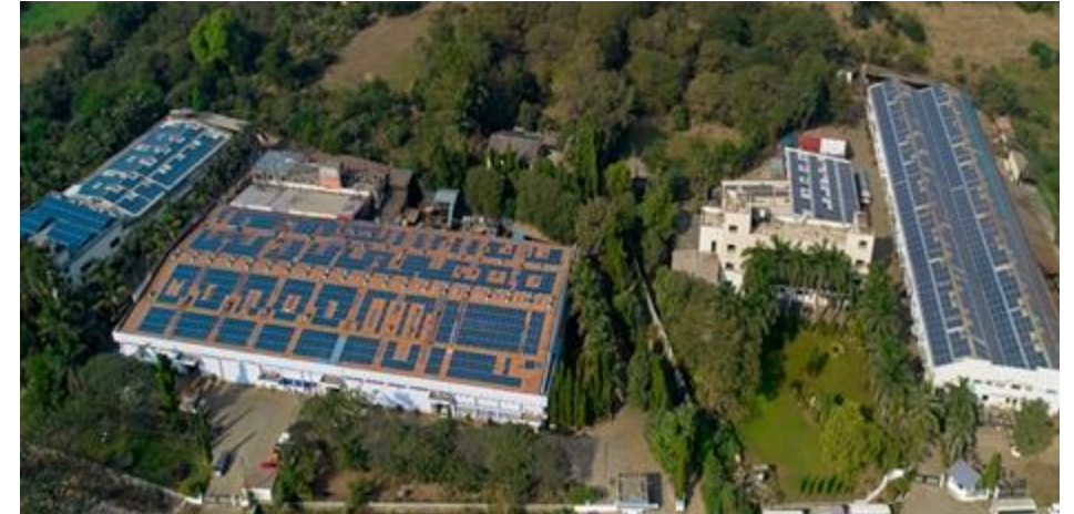
EXISTING WADA PLANT, NEAR MUMBAI, MAHARASHTRA
