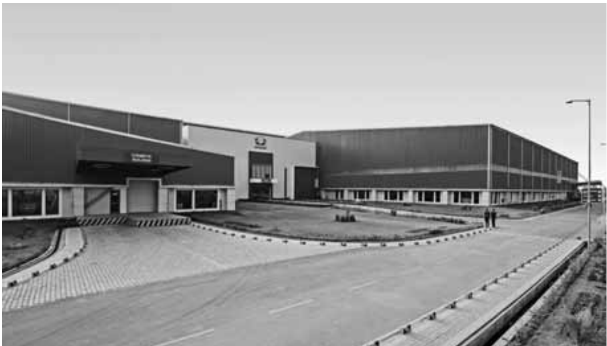
Emami's newly commissioned Pacharia plant, Guwahati, Assam
