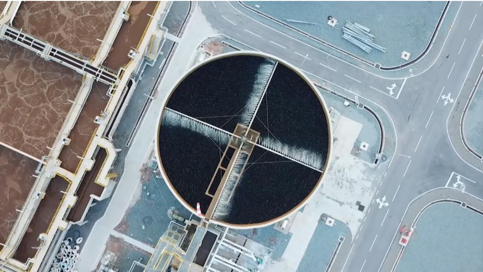
Refinery and Petrochemical Integrated Development Project (RAPID), Pengerang, Johor, Malaysia
