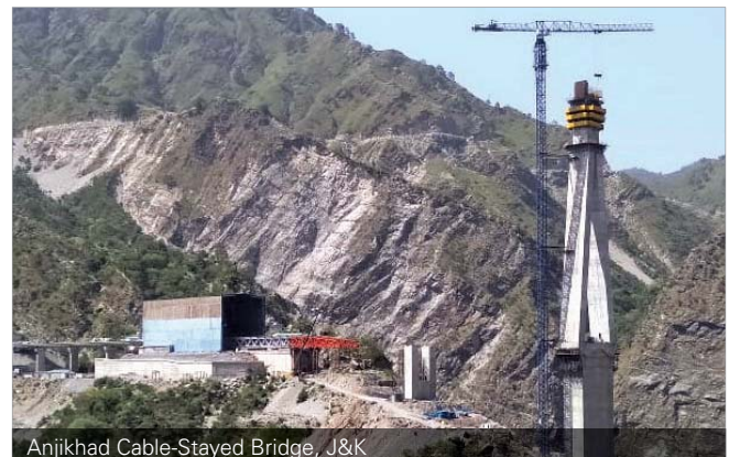
Anjikhad Cable-Stayed Bridge, J&K
