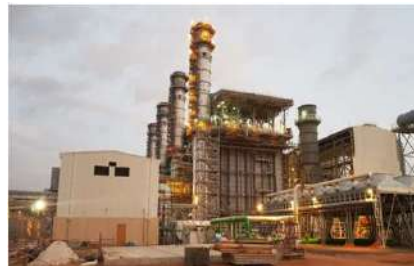
1,390 MW Waad Al Shamal ISCCPP, GE, KSA
