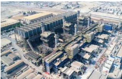
1,800 MW Alba PS5 CCPP, Bahrain (Completed Project)
