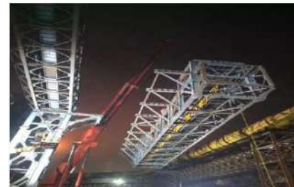
Utility Corridor, Gallery Erection, Dolvi, JSW
