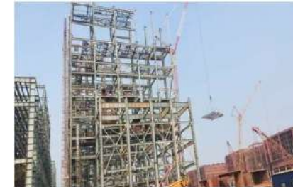
5x800 MW Yadadri TPP, TSGENCO
