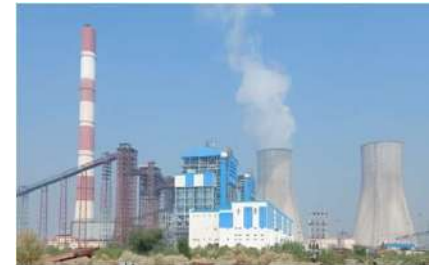
2x660 Mw STPS, Suratgrah - RRVUNL
