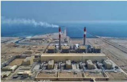
4X660 MW Shuqiaq SSPP, KSA (Completed Project)
