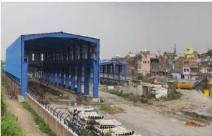
MEMU Shed at Kanpur-RVNL
