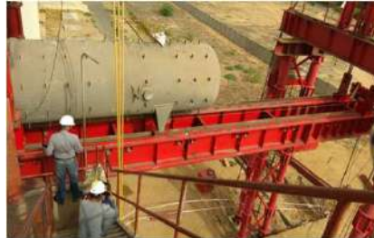
HP Heater Replacement 800 MW, CGPL Mundra 2
