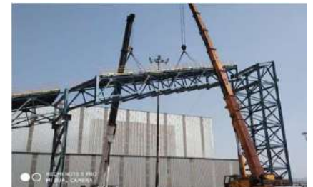
Erection of P&N Gallery at Bellary, JSW
