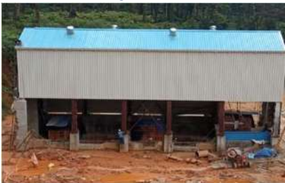
Implementation of Hydro Electric Project (2MW/5.14 Mu)-KSEB
