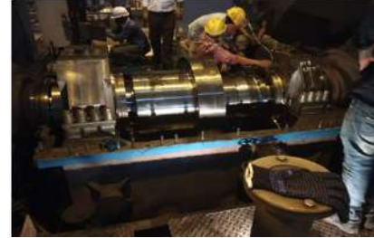
Bearing Disassembly At NTPC-Simhadri
