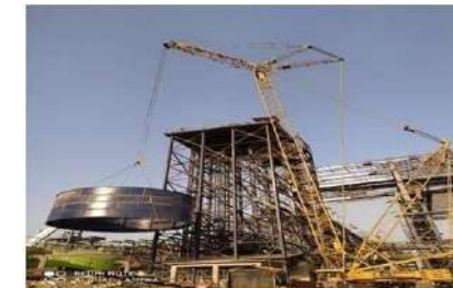
SMS II - Overhead Tank, Dolvi - JSW
