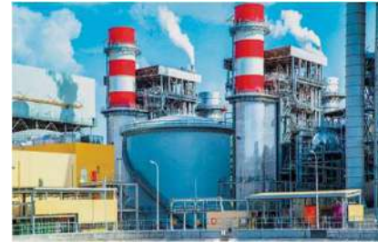
1,516 MW IBRI IPP, SEPCO – 3, Oman (Completed Project)
