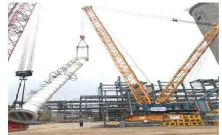
Urea Reactor Tank Installation At Ramagaundam, Telangana
