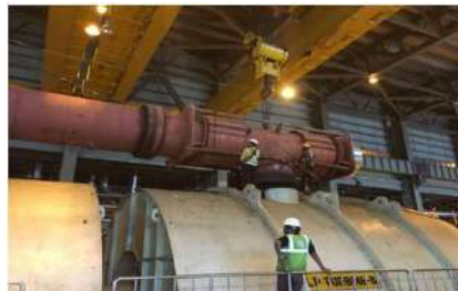
Turbine AOH, 600 MW, Udipi
