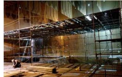
Cuplock Scaffolding Erection 800 MW, Mundra
