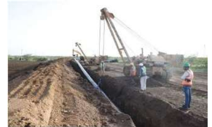
Lowering of Pipe Section, Mundra, Adani
