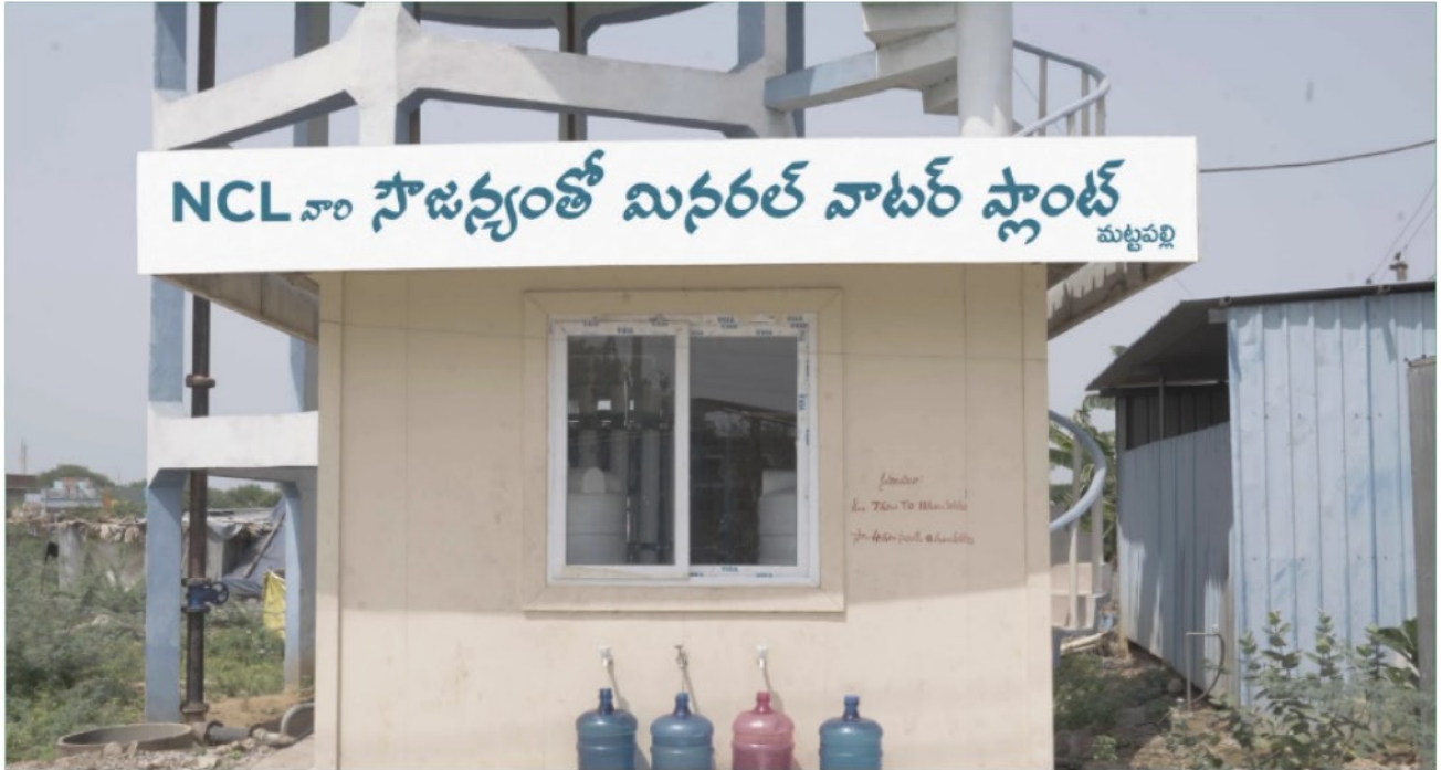
RO Water Plant
