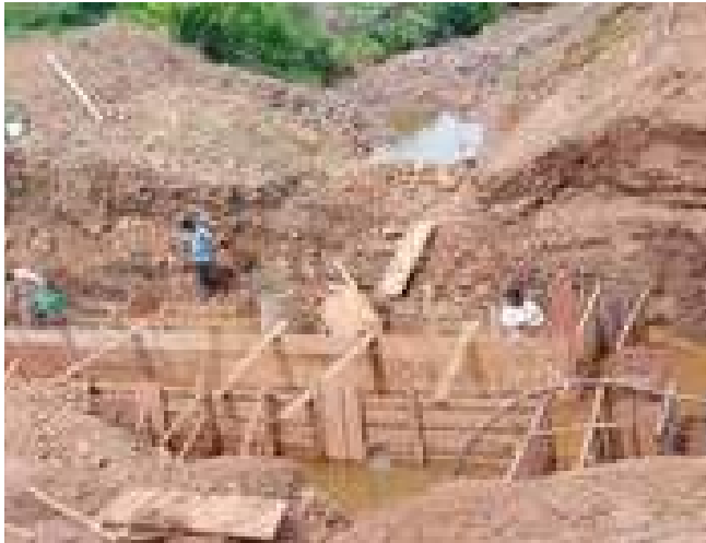
● Construction of mud dam
