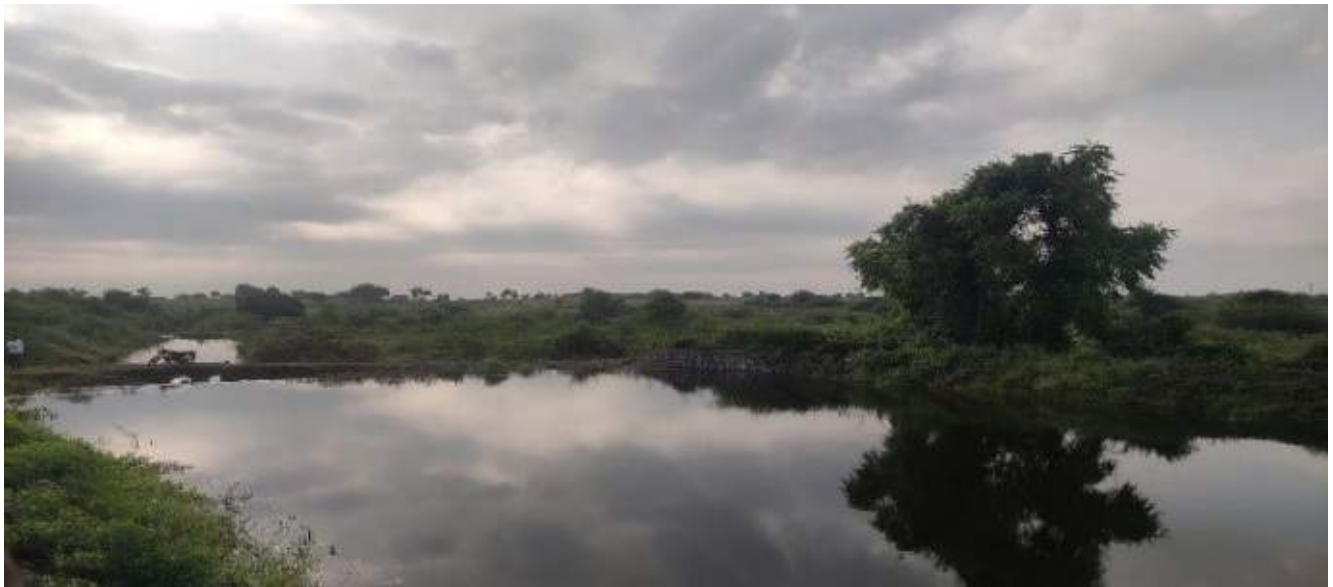
● Mud dam for storing water and percolation to nearby cultivation land
