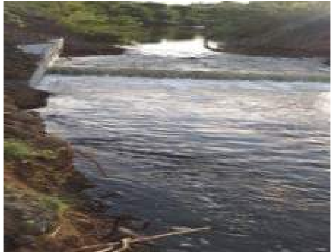
● Cement dam at Chowdary wasti Khor
