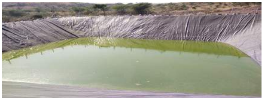
● Artificial captive water tank
