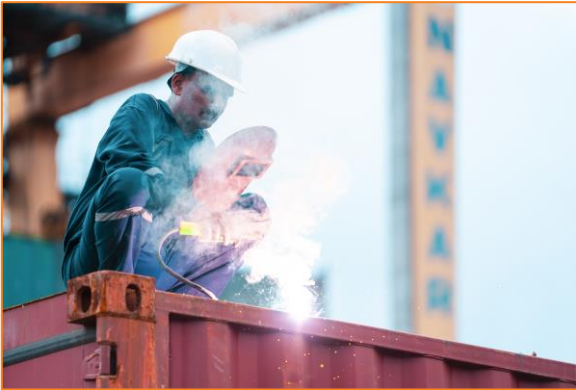
Container's repair and maintenance
