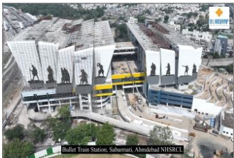
NHSRCL – Sabarmati Station
