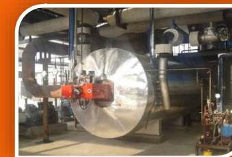
3.5 MW Thermal Oil Heater for Biscuit Baking
