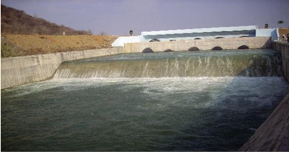
Kalwakurty Lift Irrigation Project, Andhra Pradesh
