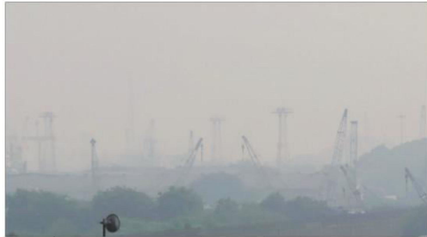
Winter is far away, but construction dust has worsened air quality.
