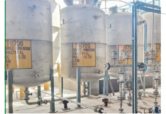
Reactor Installation Completed
