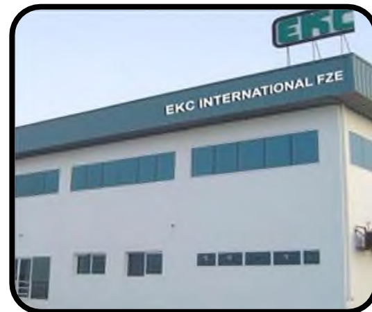
Plant II – Dubai
