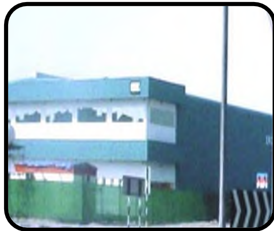
Plant I – Dubai
