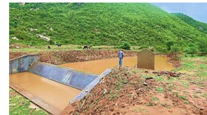
Water Conservation Project
