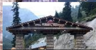
Atal Tunnel, India
