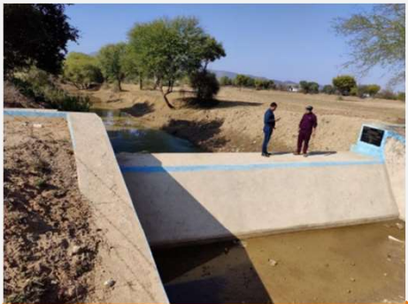
Madawari Wala Check Dam
