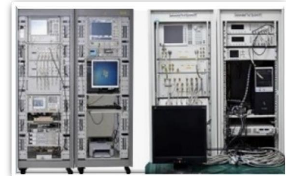
ATE ATS - Facility
