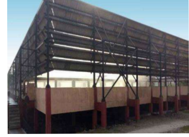
Mist Cooling System
