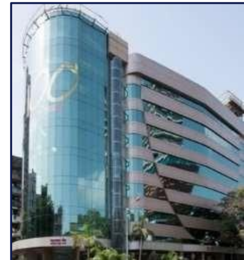
Saraswat Bank Bhavan Phase I : Upto 7 th floor
