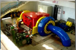
Hydro Turbine Generator & Site Installation
