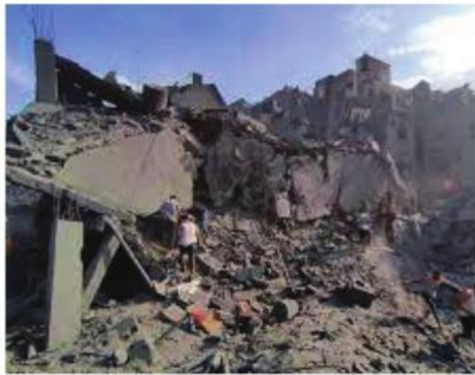
Aerial view of a destroyed building in Gaza, showing the extent of damage from Israeli airstrikes.
