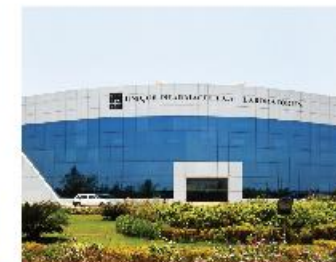
Formulations manufacturing facility at Panoli, Gujarat
