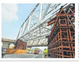
minutes before the targeted time of 5pm. The successful launch of the girder, weighing 250 metric tonne, over the Pune-Mumbai Expressway was achieved with utmost precision and adherence to safety protocols," he
