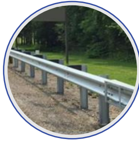
Metal Beam Crash Barrier
