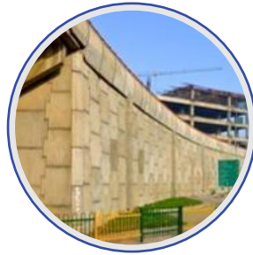
Reinforced Earth Walls
