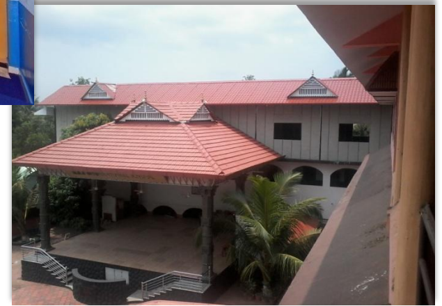
Roof Top Extension - (V-Panel )
