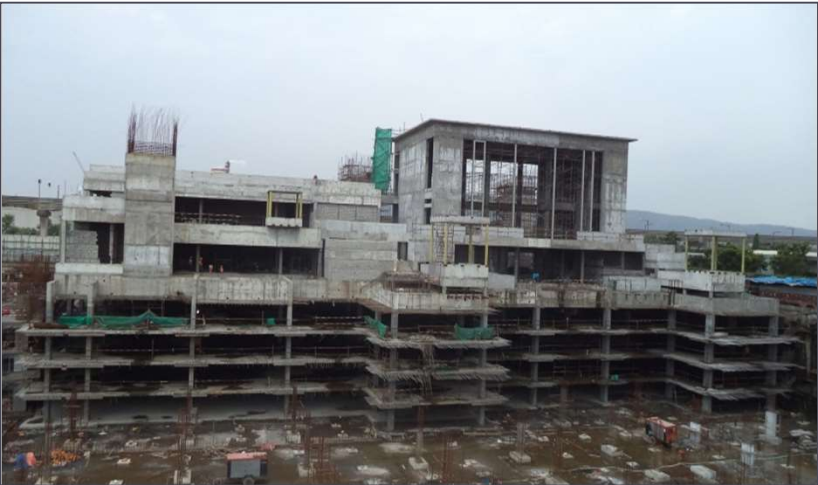
Civil Works Wadala
