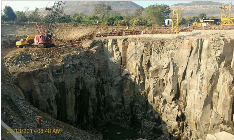
Bhama Ashed Water Supply Project
