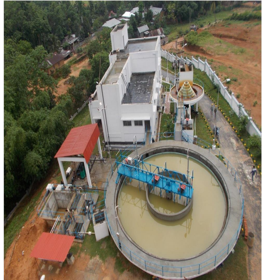
Agartala WTP project
