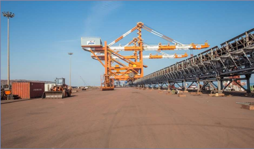
Piling & Civil Works for JSW, Jaigad
