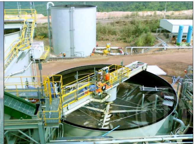
HDPE Tailing and Decant Piping Installation
