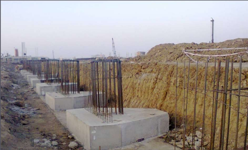
Foundation BASF, Dahej
