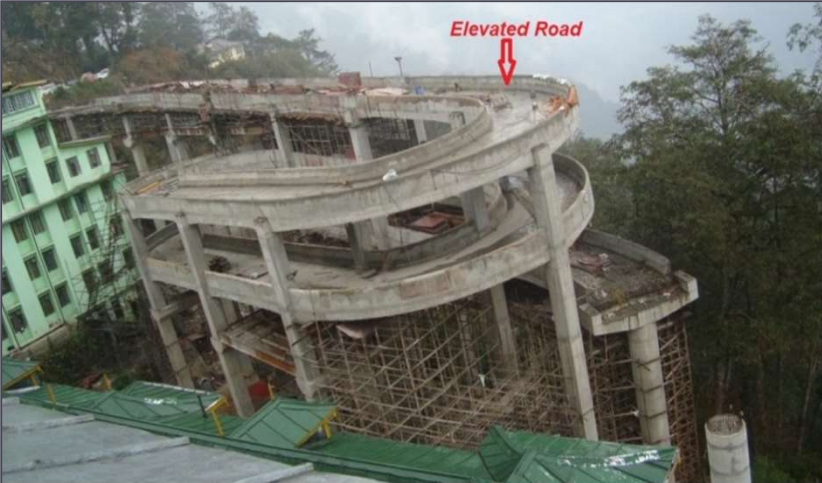
Piling & Civil Arctech, Gangtok
