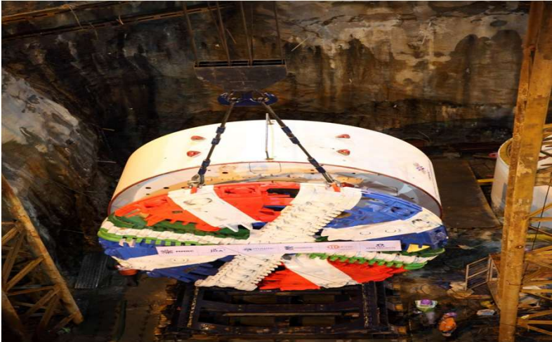
Lowering of TBM, Mumbai Metro L3
