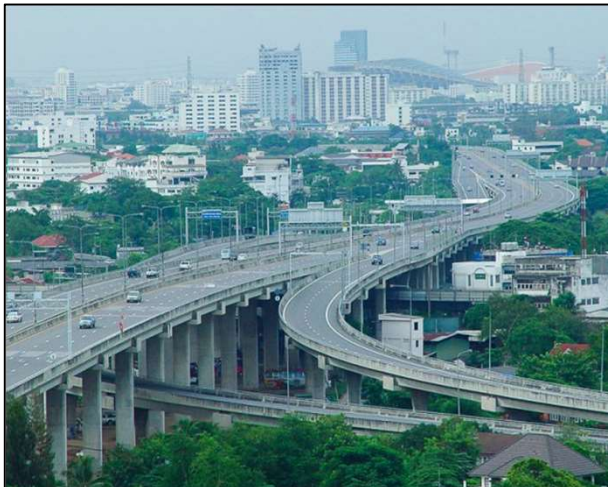
Ramindra - At Narong Expressway System
