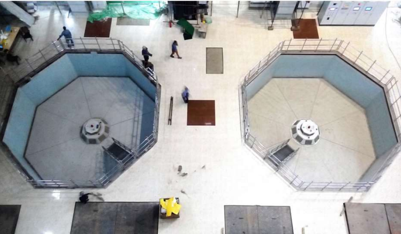
Power House, Umtru
