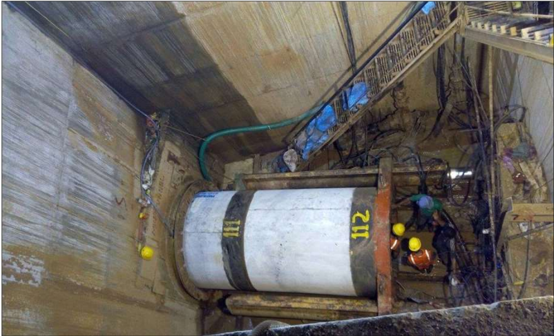
VMSS – Micro Tunneling Vadodara
