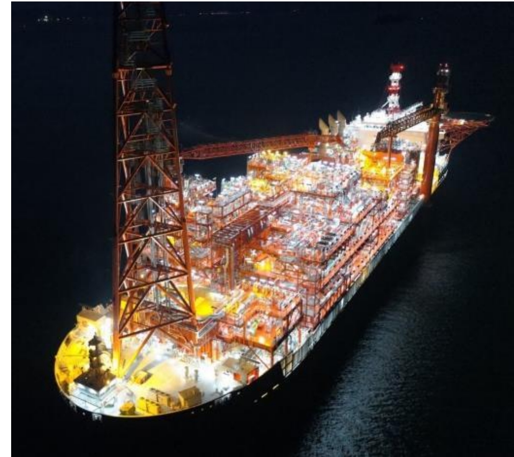
FPSO Installed and Commissioned
