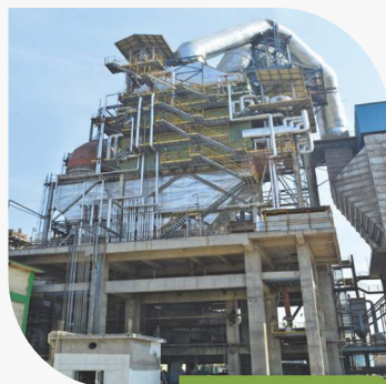
WHR at Narsingarh Plant
