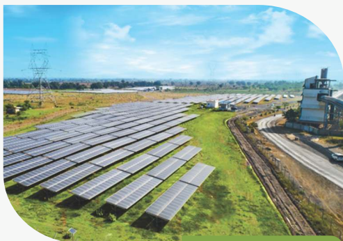
Solar Power at Damoh
