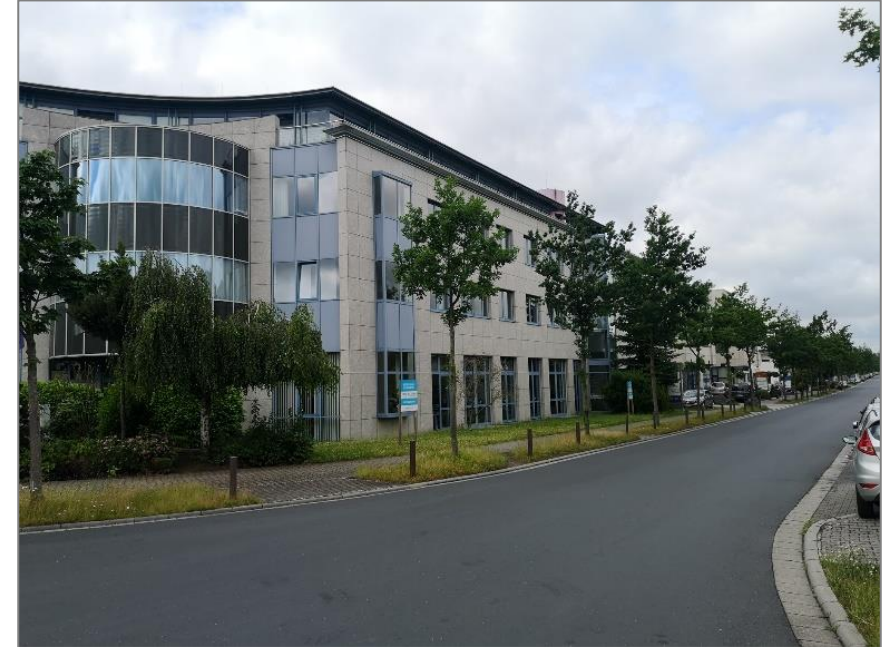
R&D Office, Germany
