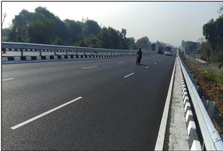
Pune Satara Road Project
