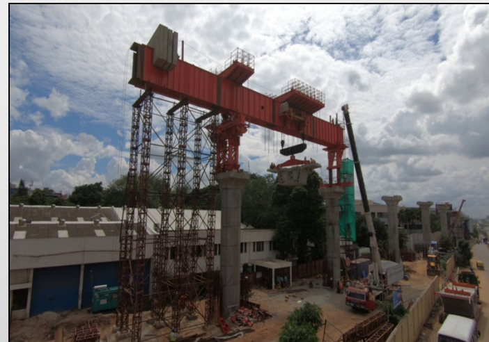
Bangalore Metro Project
