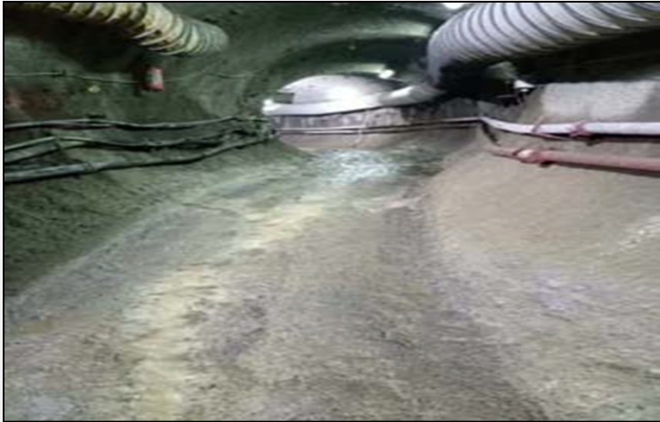
Underground Kolkata Metro Project
