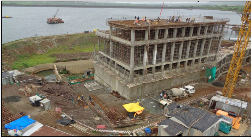
Bhama Ashed Water Supply Project
