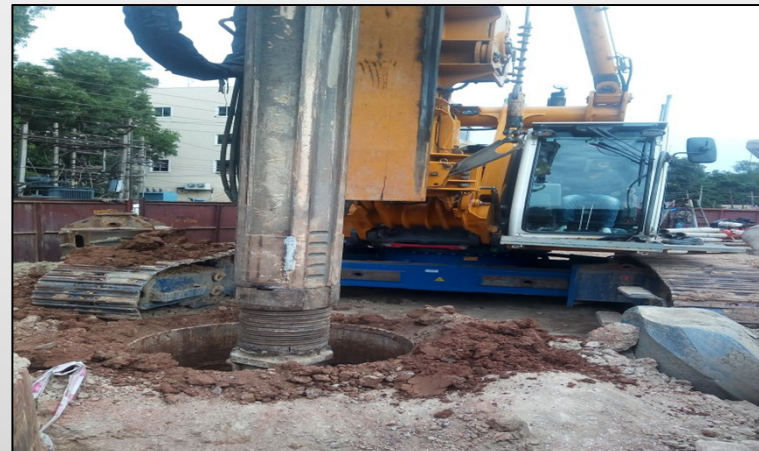
Piling Work at Bangalore Metro
