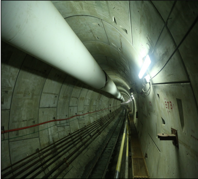
Mumbai Metro Underground Tunnel Project
