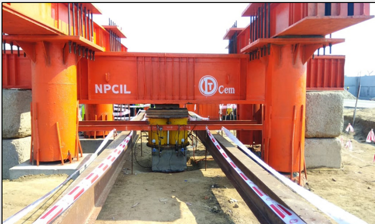
Ground Stabilisation work for Nuclear Power Corporation
