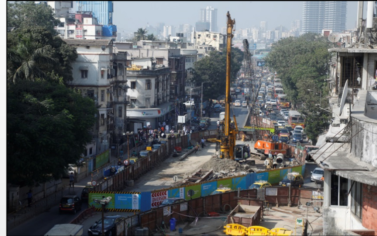
Piling Work at Mumbai Metro
