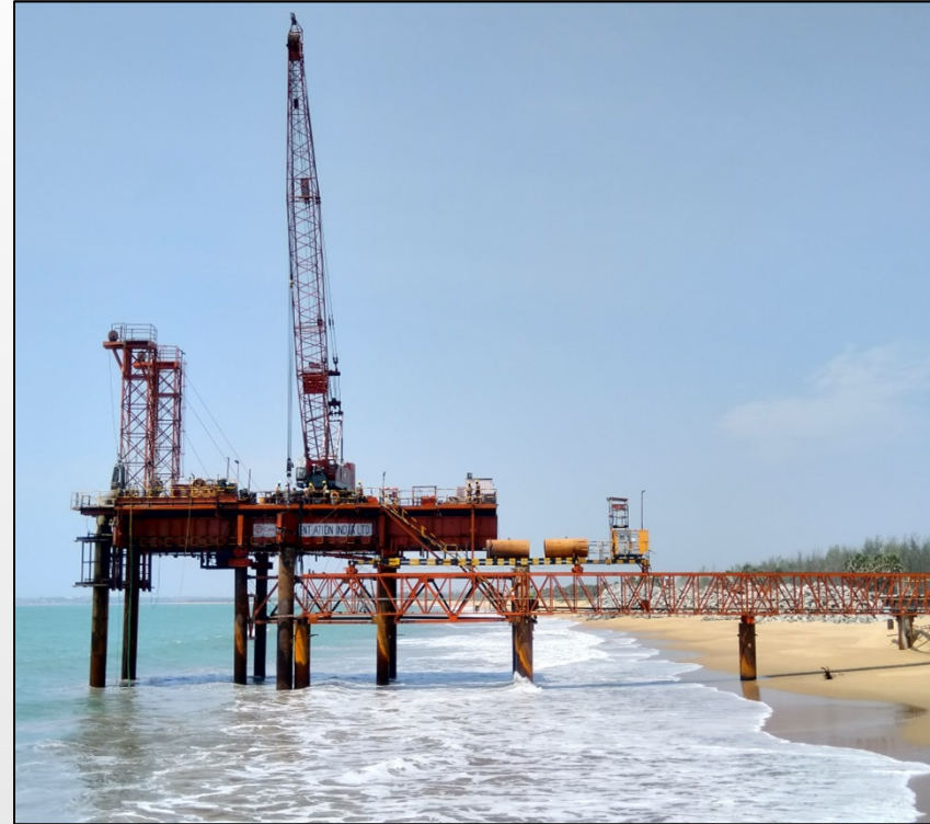
Udangudi, Tamilnadu Power Project
