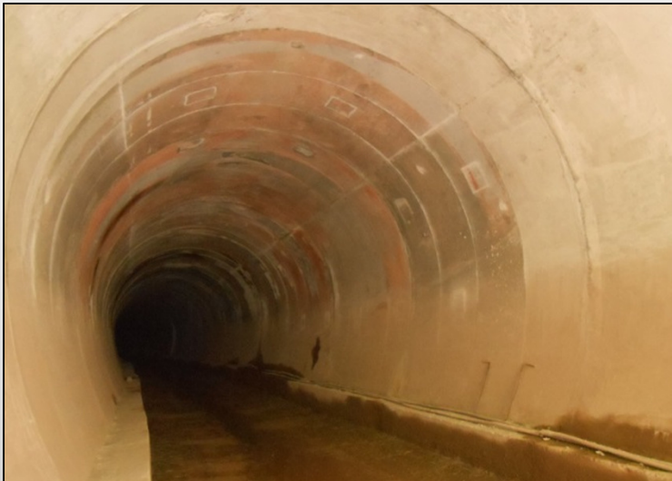
Tunnel for Indian Railways
