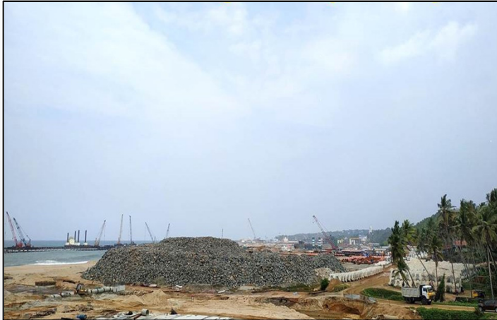
Vizhinjam Break Water Project
