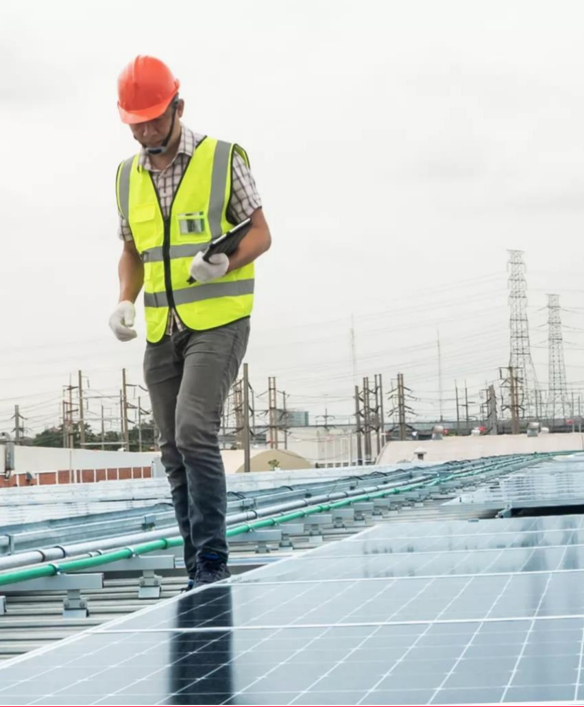
Grid connection for upcoming 300MW solar PV power plant in Bikaner, Rajasthan
