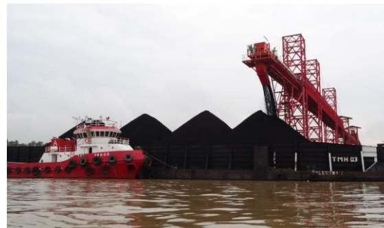
Coal Being loaded onto Barge via Conveyor at Jetty
